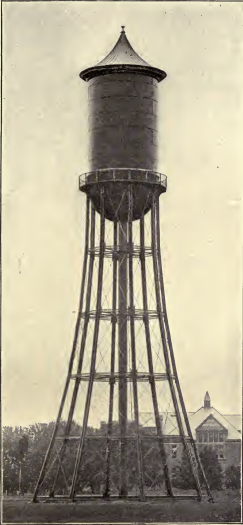
FIG. 62.—AMES, IOWA, STEEL WATER-TOWER.
